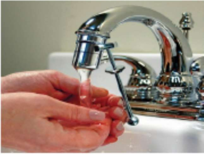
Photographs: Spring loaded push taps
